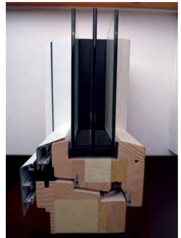
Section through a typical Passivhaus-suitable triple-glazed window, in this case with an aluminum finish externally and wood internally.
